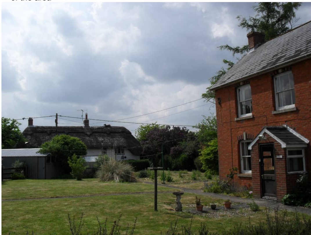
Fairview, as existing – Gaddon House in rear of picture
